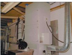
Figure 18 Dust extraction at flour sack-tip point
