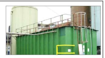
remained in the tank, resulting in heavy corrosion which affected the oxygen level; this should have been 20.9% and it was in fact 4%. The employees only entered the tank after carrying out pre-entry checks and then selecting and using the appropriate equipment. This prevented a fatality.
