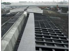
Figure 6 Walkway and fallboards on fragile roof
